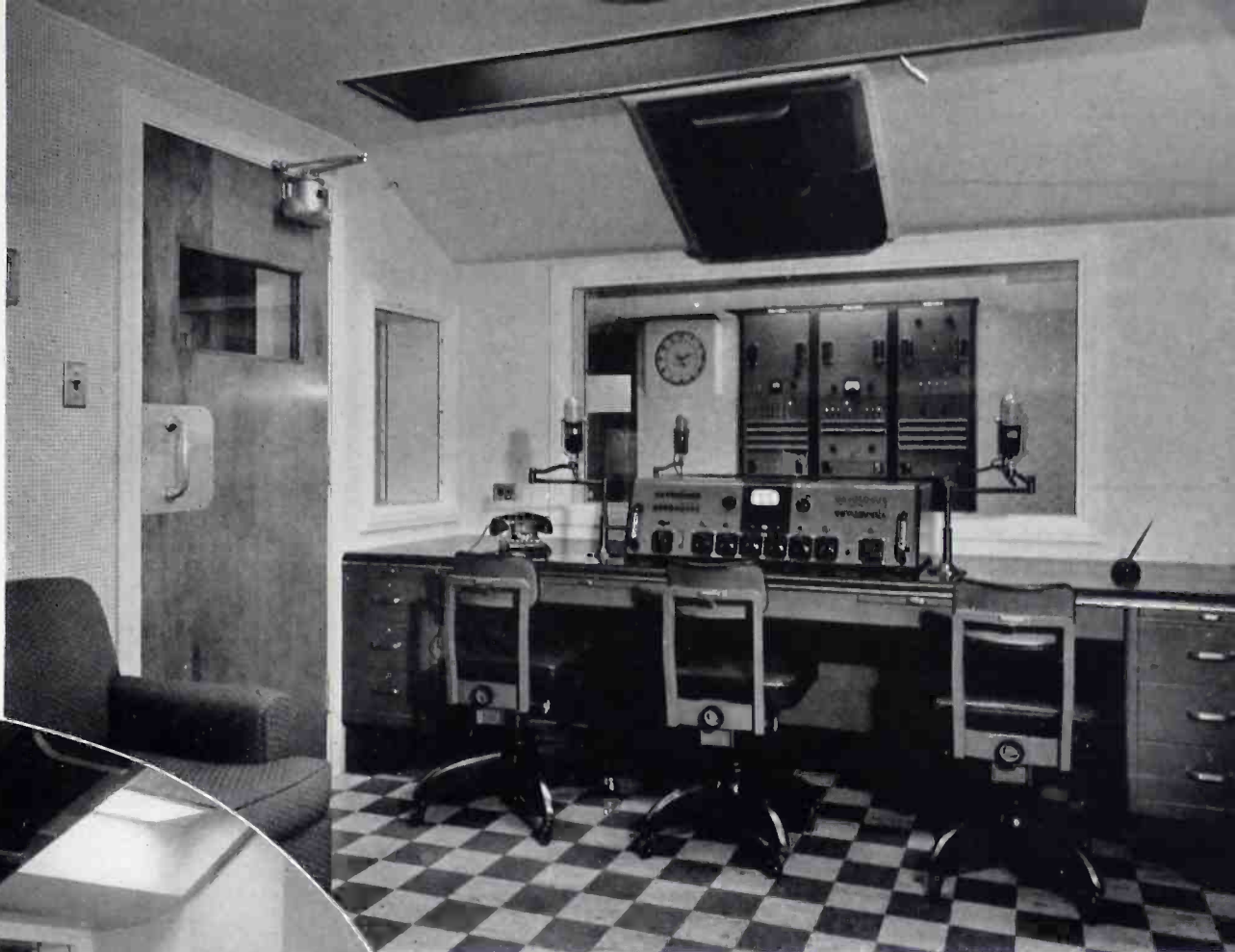
▲ Control Room for Studio B is provided with two announce positions and an RCA 76-B1 Console. The Studio C Control Room and Master Control Racks may be seen through the window.
